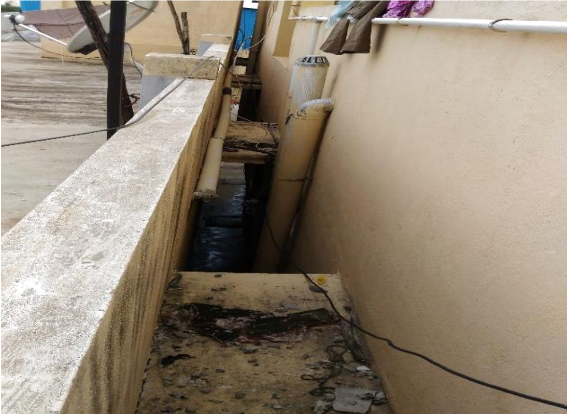
Photo showing in between the building - 1
