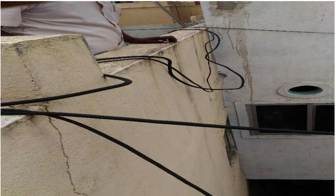
Photo showing on the North side of the building
