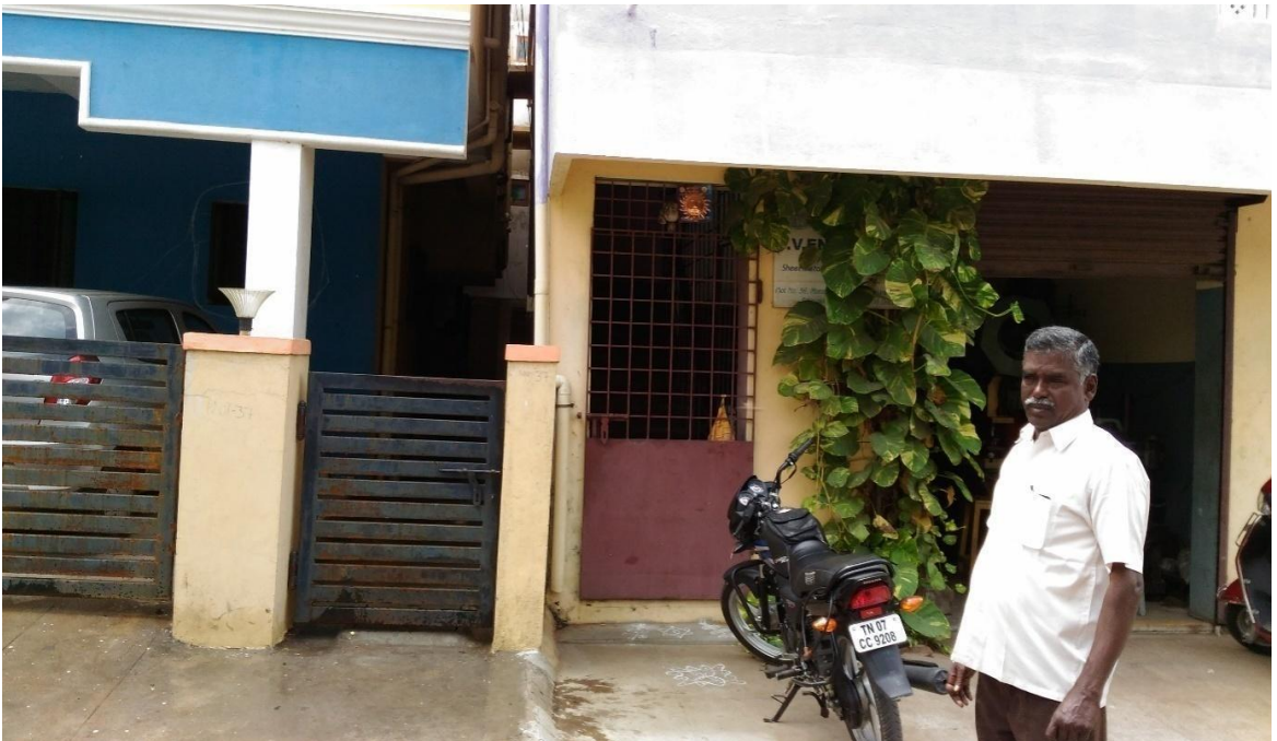
Front portion of the Building
