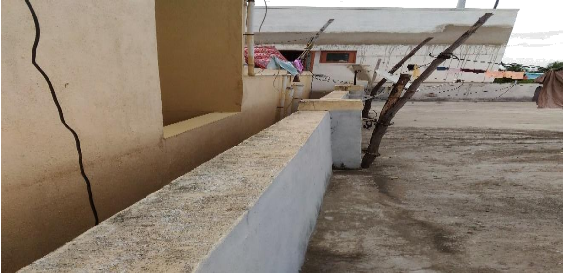
Photo showing the tilt in terrace floor -1
